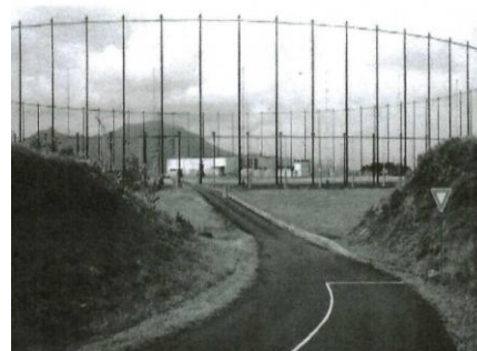
Circularly Disposed Antenna Array (CDAA) built for HF monitoring & direction finding. Wahiawa, HI
