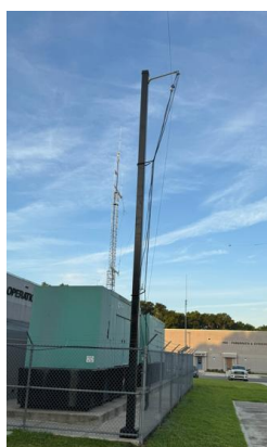
New hurricane-rated Tower supporting OCF type HF antenna
