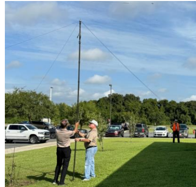
(Photos L&R) MERT members constructing the 40/80 Meter NVIS antenna MERT owns on July 17 th .
