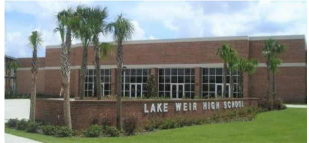
Lake Weir High School – A MCPS Shelter facility.
