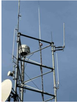
Photo of tower before having old antennas and cables removed.
