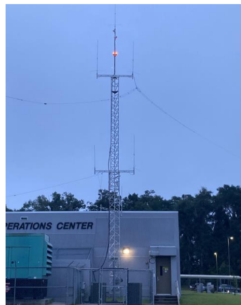
MERT's Tower at the EOC was inspected early Wednesday Sept. 27 th for proper light operation. It passed!
