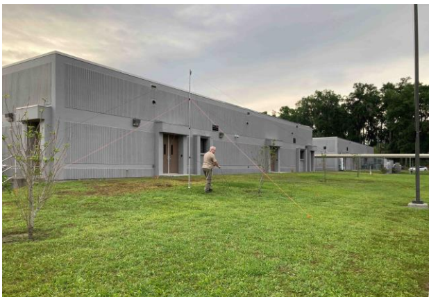
NVIS antenna installation completed and ready.
